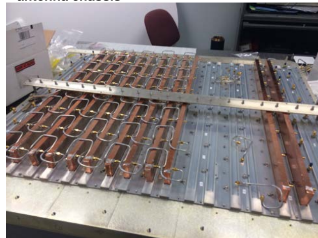
Installation of 45 mm wide feedboards on antenna chassis
