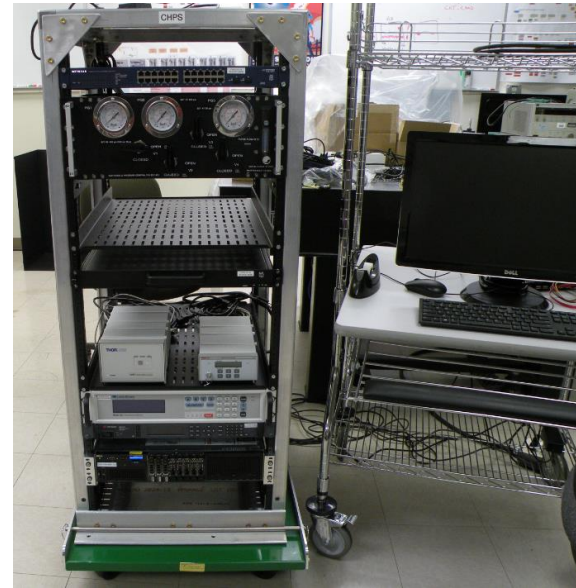
GN2 Purge and Pressure Control System and CHPS Equipment Rack
